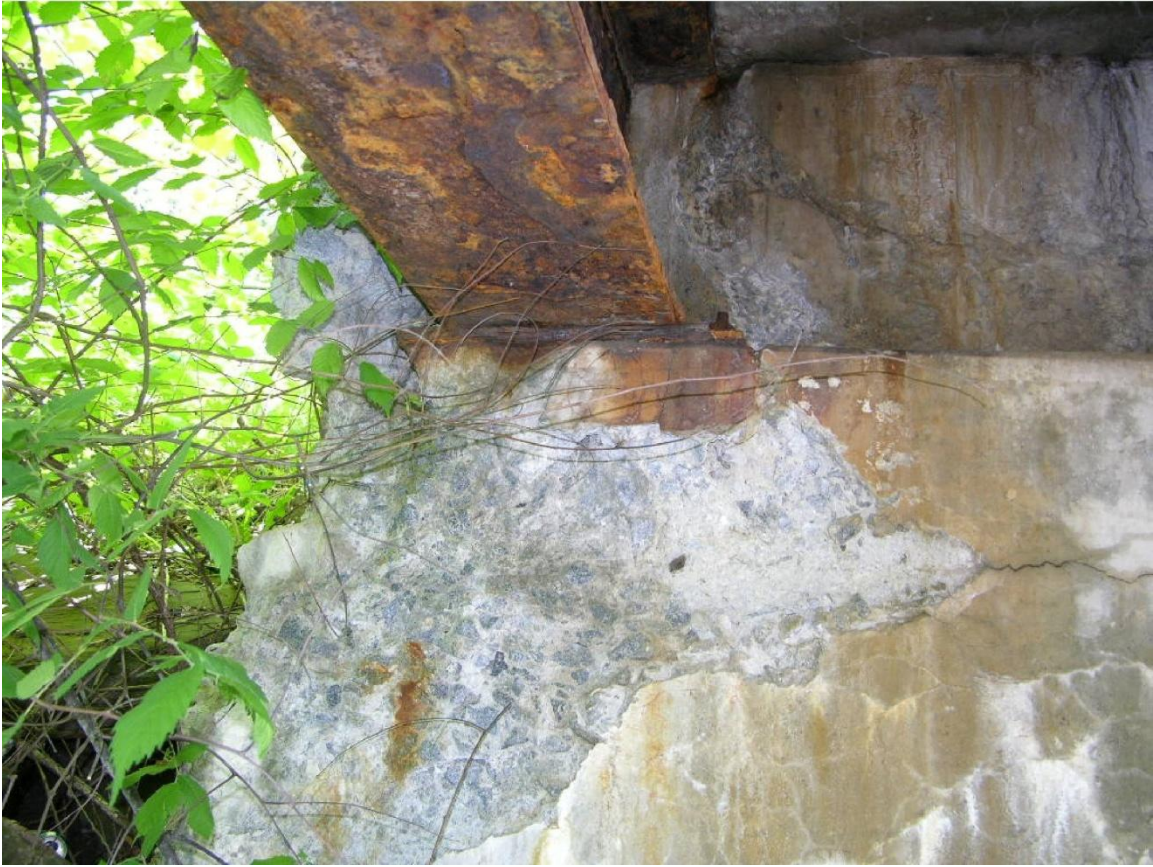
Abutment Deterioration
