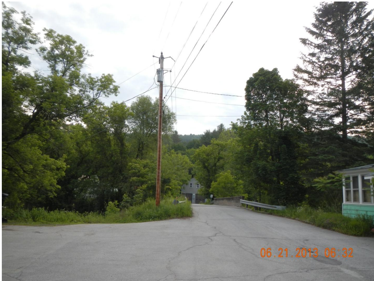
Figure 3. View of existing site. Photograph was taken facing east.
