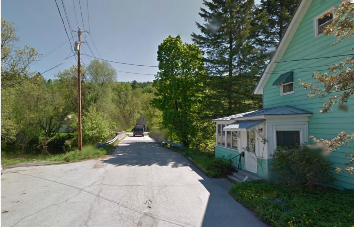
Looking east over the bridge at the narrow roadway
